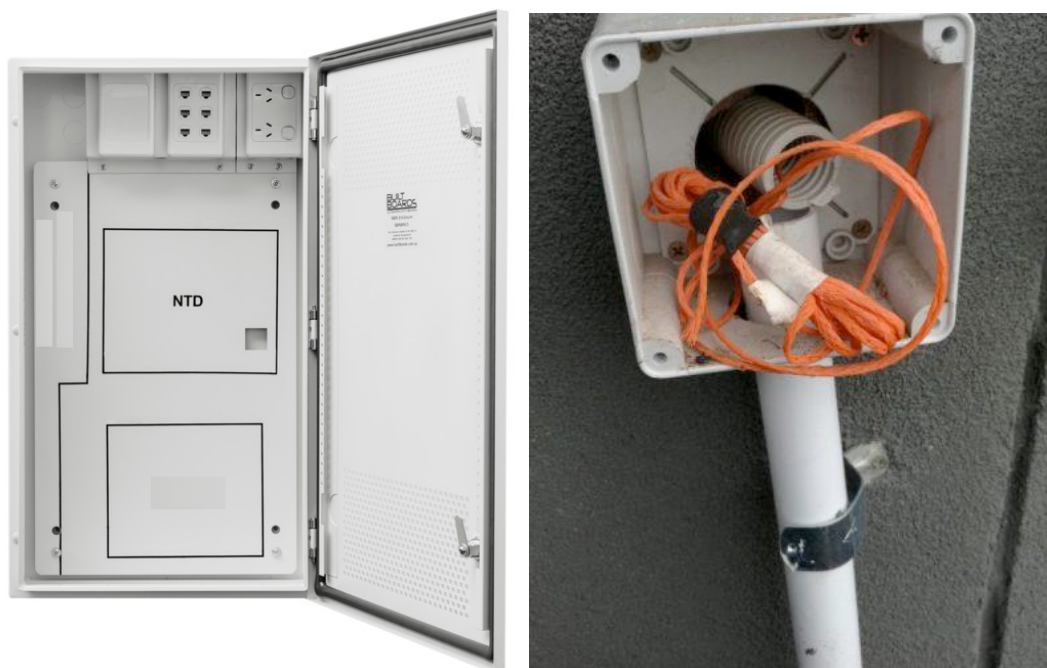
Picture 2 - Required cabinet setup and Junction box setup with drawstrings
